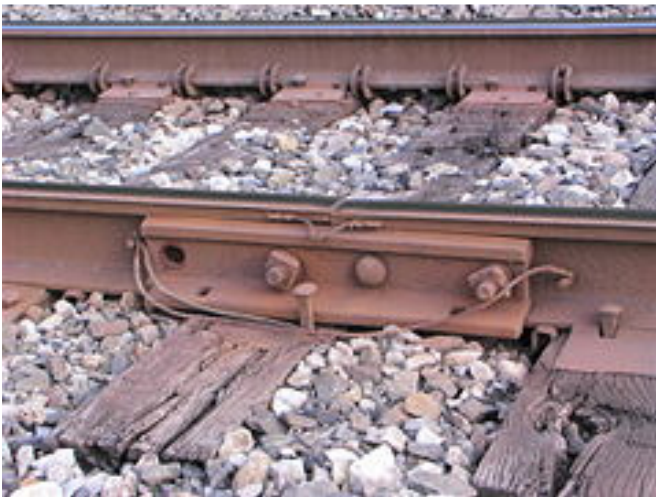
Joint court de la Pennsylvania Railroad
